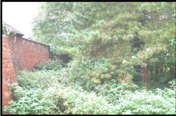
Existing route near point A (2007)
